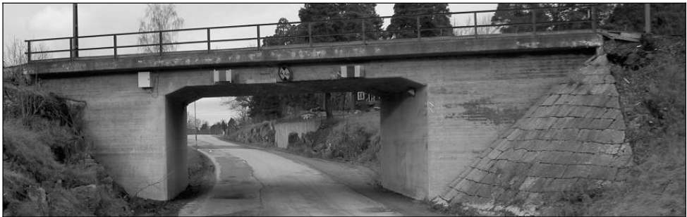
Figure 7.3 Photo of the Frövi Bridge southern face
